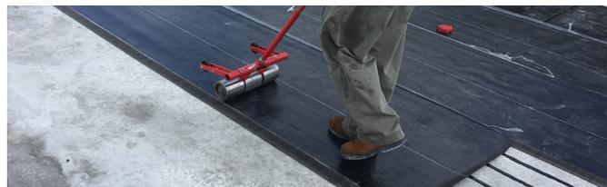
Side laps and end laps may be addressed by using beads of COLPLY EF dispensed from cartridges or may be heat welded. If using COLPLY EF in the laps, ensure enough adhesive is applied for a  $\frac{1}{8}$ " to  $\frac{1}{4}$ " bleed out from the lap.
