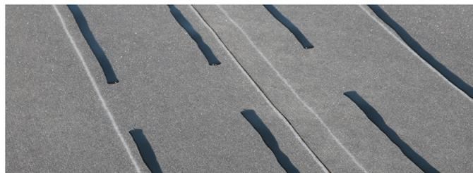
Once the adhesive is applied in ribbons, the membrane must be immediately applied. After rolling out the membrane into the adhesive, a weighted roller should be used over the entire surface of the membrane. The weighted roller is critical to ensuring proper bead width of 2  $\frac{1}{2}$ " to 3" beneath the membrane.
