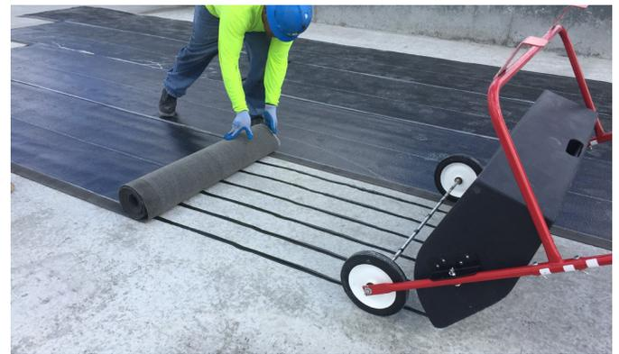
When using the spreader cart to apply COLPLY EF in ribbons, 3/4" to 7/8" inch holes should be predrilled for the required spacing (12" o.c., 6" o.c., etc.). With the cart laying down, up to four pails of COLPLY EF can be loaded into the tank at one time (20 gals). With an application rate of 1 gallon per square, 1 full tank will cover between 15 and 20 squares.
