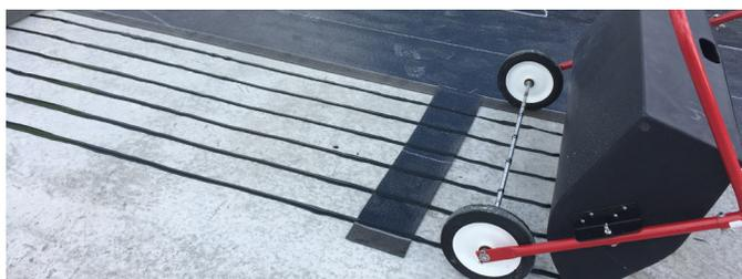
After 30 to 45 minutes of application (may be less based on heat and humidity), any adhesive left in the tank will begin to skin over. Once this happens, this tank cannot be refilled and must be swapped out for a new tank. Multiple tanks should be kept on site at all times.
