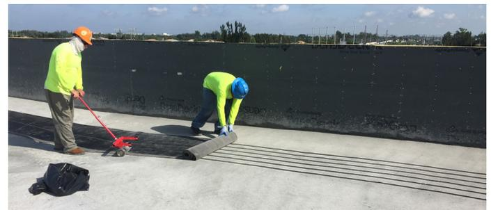
To apply, simply turn the cart over and begin walking in the direction the membrane will roll out. Be sure to maintain the proper bead size of 1/2" to 3/4" while applying. Every 33 to 45 feet, a six inch horizontal break must be provided to allow for cross venting between channels.
