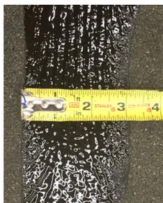
The cartridges are then ready to be inserted into the battery applicator and applied. Be sure to maintain the proper bead size of  $\frac{1}{2}$ " to  $\frac{3}{4}$ " while applying. Every 33 to 45 feet, a six inch horizontal break must be provided to allow for cross venting between channels. Prior to application of the adhesive, cut 6" scrap membrane pieces. These can be placed on the deck and removed once the adhesive has been applied, creating a gap with no adhesive.
