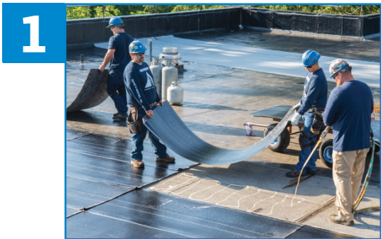
Place SOPRASMART system in desired position.
