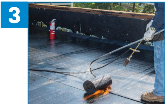
Roll self-adhered portion of Duo Selvedge side lap and then heat weld remaining 60%. Apply SOPRALENE FLAM 180 Cut 13" cover strip over all end laps.
