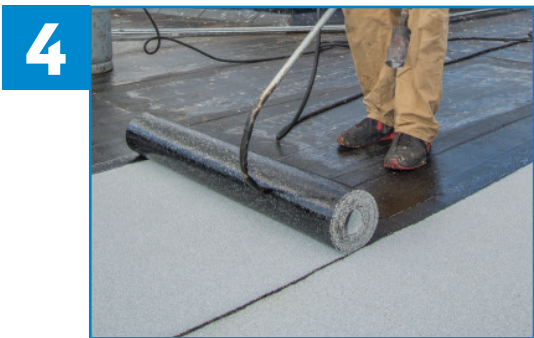
Subsequent membranes are installed by heat welding, cold adhesive, or self-adhesive applications
