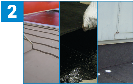
Install SOPRASMART system with mechanical fasteners or DUOTACK 365 adhesive.
