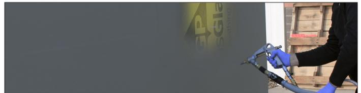
Once the application is complete, inspect the wall for any blisters, holes, or areas in need of repair. Apply additional SOPRASEAL 202 or 203 to these areas. Allow to dry completely, typically 2-4 hours at 77°F (25°C) and 50% relative humidity. Exposure of SOPRASEAL LM 202 or 203 to the elements is not recommended past 180 days.
