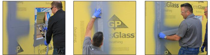
If spraying, there is no need to wait for the surface to dry. \*\*SOPREMA recommends the use of low pressure, high-volume spray equipment capable of a pressure range above 40 psi. Coat the field of the exterior sheathing or plywood and recover the seams, corners and joints. If deemed necessary, a second coat may be applied after checking to ensure that the surface is free of voids, holes or blisters, all repairs are completed, and the initial coat has dried.
