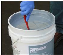
The substrate should be clean, sound, free of excess water and loose materials, grease and any contaminants, which may compromise the performance of the product. Do not apply to frozen or frosted substrates.
