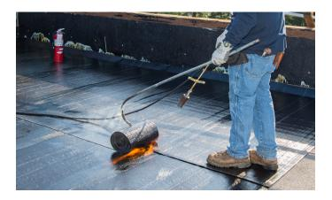
To seal film surfaced end-laps via heat welding, weld the SOPRALAP™ FLAM or SOPRALAP SP strip-in plv. centered along the end joint.
