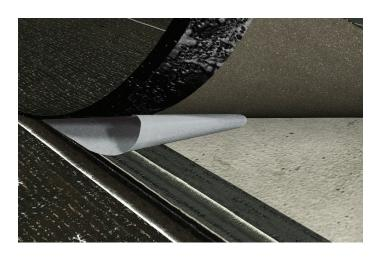
During installation, ensure the DUO SELVEDGE side-laps are maintained clean and dry with the self-adhesive release fiilm applied. To seal the side laps, remove the self-adhesive release film from the DUO SELVEDGE side lap and apply pressure with a weighted roller. Heat-weld the remaining outer edge of the SOPRASMART side-lap to ensure the sidelaps are sealed watertight.
