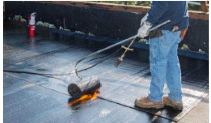
To seal film surfaced end-laps via heat welding, weld the SOPRALENE® FLAM 180 Cut 13" or SOPRALENE® 180 SP 3.0 Cut 13" strip-in ply, centered along the end joint.
