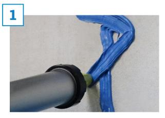
Prior to spraying SOPRASEAL LM 204 VP, prepare all sheathing joints by applying a thick monolithic bead of SOPREASEAL Liquid Flashing into the joint. Create a zigzag pattern over the joints with a minimum of 2 inches of coverage.
