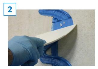
Spread the SOPREASEAL Liquid Flashing membrane with a trowel to acheive a monolithic flashing at a minimum of 20 wet mils, free of voids or pinholes. Allow product to skin prior to spraying.
