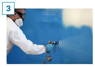
Apply SOPRASEAL LM 204 VP to the desired thickness directly to the prepared substrate.
