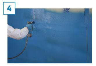
Allow to dry completely. Temperature and humidity levels will influence the curing times of the SOPRASEAL LM 204 VP. Typically, the membrane is tack free in 60 minutes at  $70^{\circ}$ F ( $21^{\circ}$ C).
