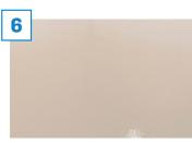
Finished surface. No further sealing is necessary. The area is trafficable and can be returned to regular service after one hour.
