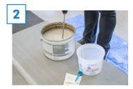
Thoroughly mix the resin and color additive in the bucket for 2-4 minutes.
