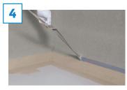
Immediately back roll with a dry roller to even out the application. Then remove the masking tape.
