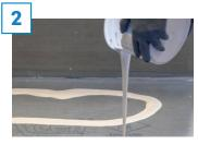
Pour catalyzed resin onto the prepared substrate. Provide sufficient material to cover the surface. Consult the product specifications for project coverage rates.
