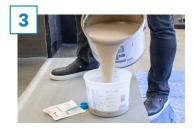
For batch mixing, pour off colored product into a clean mixing bucket.
