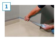
Before mixing materials and starting any work, ensure the area is clean and dry. Prepare and mask off application areas with masking tape.
