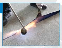
If necessary, cover the SOPRAJOINT PLUS with a cap sheet membrane centered over the joint and fixed on one side or with another mechanical protection.
