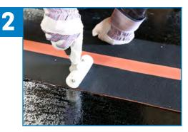
Apply pressure on the SOPRAJOINT PLUS to maximize adhesion.
