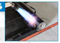
Cover the flange with a cap sheet membrane all the way up to the edge of the core and apply pressure.
