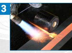
Weld a 150 mm (6 in) reinforcing strip centered on the edge of the flange and apply pressure.
