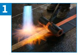
Using a propane torch, heat the base sheet and unroll the SOPRAJOINT PLUS on the liquefied bitumen of the base sheet membrane.
